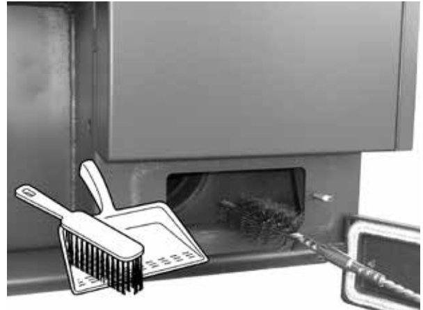
Sample cleaning of the flue way - bottom lid
